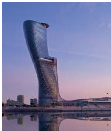
Hotel Hyatt Capital Gate, Abu Dhabi: horní sprcha Raindance® S 240 Air.
